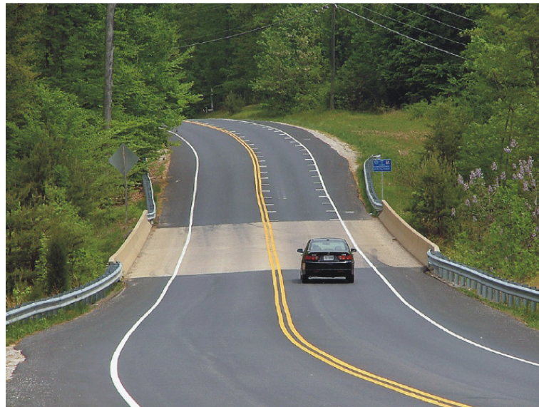
Figure 2.1 Optical speed bars (Virginia DOT)
