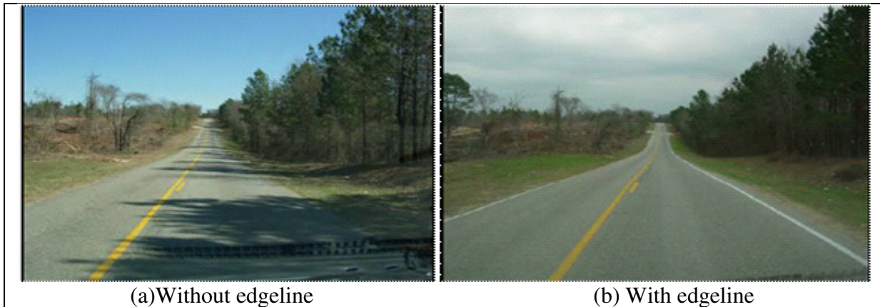
Figure 2.14 FM 15 (a) without edgeline and (b) with edgeline
